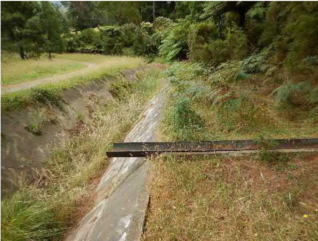
Plate 24 Surface diversion channel at O'Shannassy aqueduct (G.Vines 16/01/2019)
